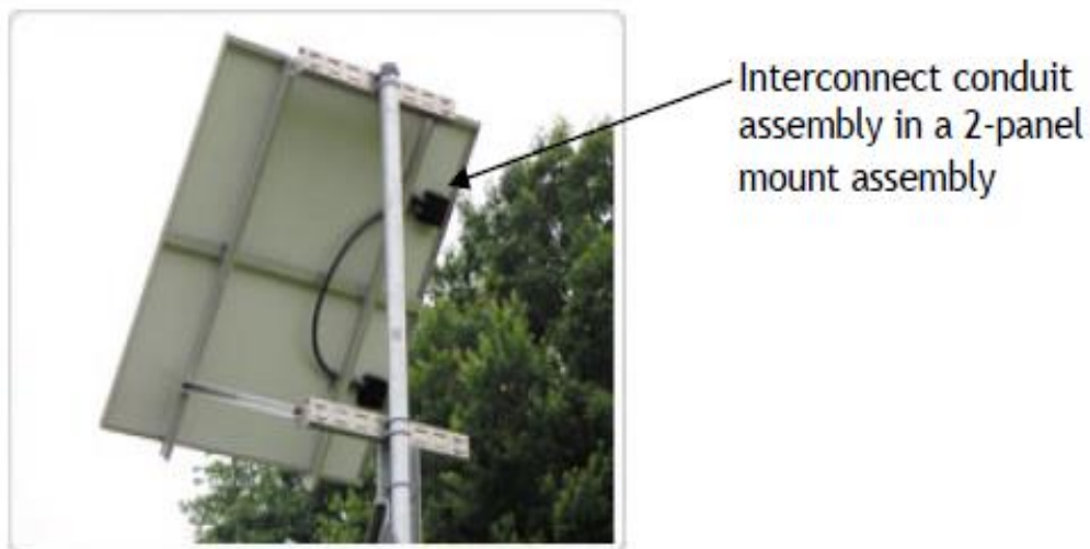
Figure 2.4: Two Module Mount with Module Interconnect Conduit Assembly
